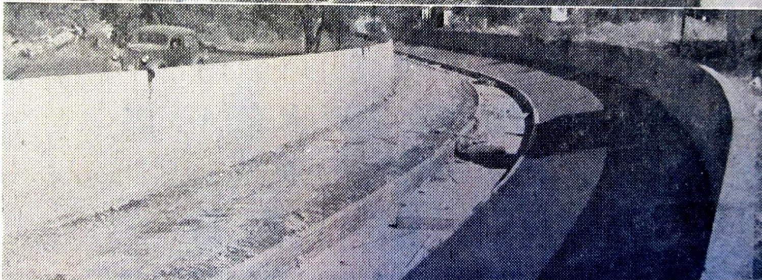
Paving of Mill creek channel is making continuous progress as the contractor, Guy F. Atkinson Co., speeds work in order to complete the job before the winter rains set in. Upper photo shows concrete being poured on one of the side slabs, which slope from the outside retaining walls down to the center trench. As can be seen, the slab is reinforced with steel throughout. In the lower picture can be seen a section in which both the center trench and south slab have been completed, leaving only the north slab to finish the job.—(Staff photos, Davison engraving).
